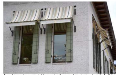
Operable awnings and shutters control how much sunlight enters the building (NW 23rd Ave and Flanders St)
