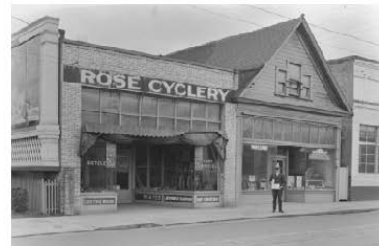
Historic photo from 1929 shows the benefits of retractable awnings and transom windows on a grey Oregon day.
