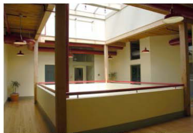
This atrium with skylight above allows light to travel deep into the building. (SW 1st Ave and Pine St)
