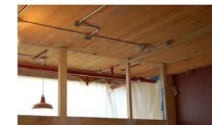
Exposing original wood ceilings adds visual warmth. Reroute windows to the ceiling allows natural light further into interior spaces
